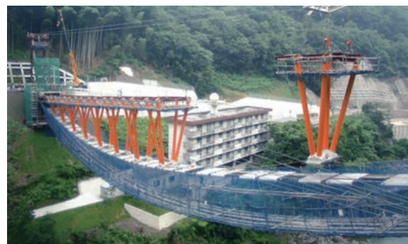
Fig. 2 Construction on suspension structure
